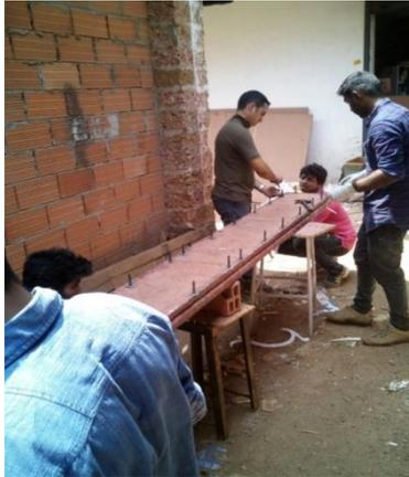
**Fig 11:** fastening male and female parts for curing
